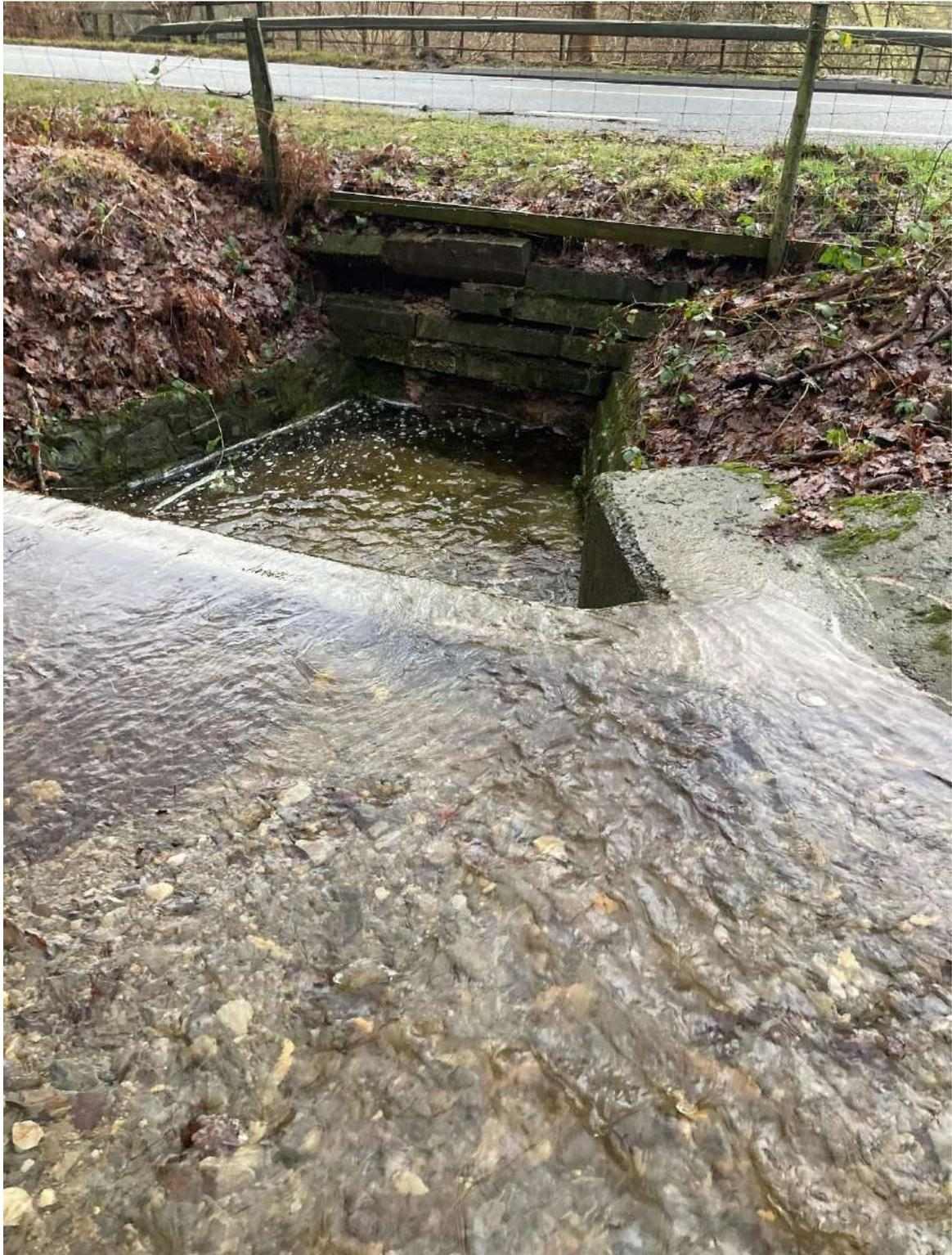
Culvert adjacent to roadside to prevent flooding from stream by holding up flow
